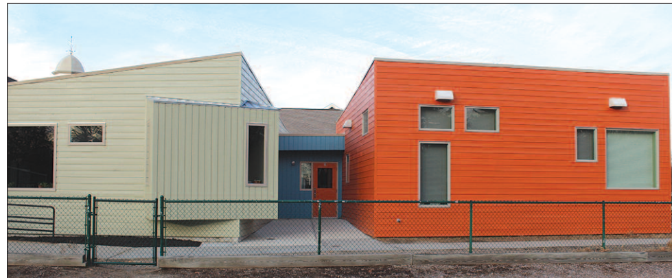
The new 6th grade classroom addition completed.
